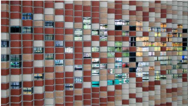
**Figure 2: Close-up of *The Digital Bricks*, containing polished translucent bricks interlaced with traditional clay bricks. All bricks are stacked at varying, predefined depths relative to adjacent bricks. Each ‘digital brick’ consists of a translucent brick with a rear-mounted high definition and high brightness LED screen that are invisibly located within the wall cavity.**
